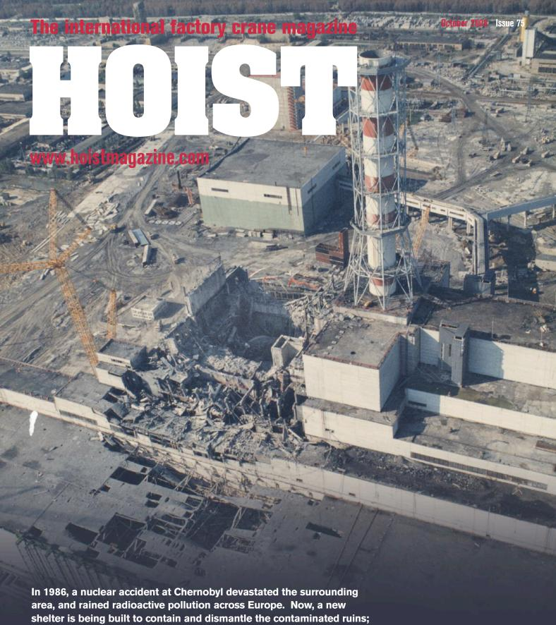
shelter is being built to contain and dismantle the contaminated ruins; within the confines of the shelter four highly customised bridge cranes will play a vital role in the clean up operation
