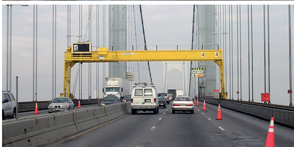
Traffic could flow under the cranes to avoid closure during construction
